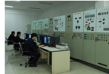
Rubber mixing microcomputer monitoring room
